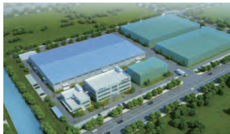
Wuxi Airthink Production Plant Phase I (Skid Intelligent Air Station, Centrifugal Compressor)
